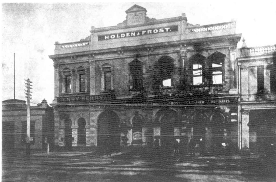
THE GRENFELL STREET FIRE. FRONT ELEVATION OF MESSRS. HOLDEN AND FROSTS WAREHOUSE.
